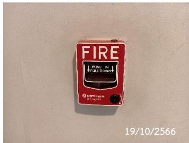
Fire Alarm Manual Station
